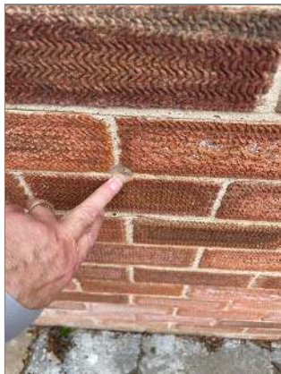
Photo - 23 Drill hole cavity insulation fitted
