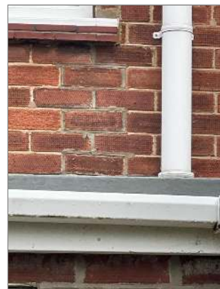
Photo - 32 Repaired cracks - rear
