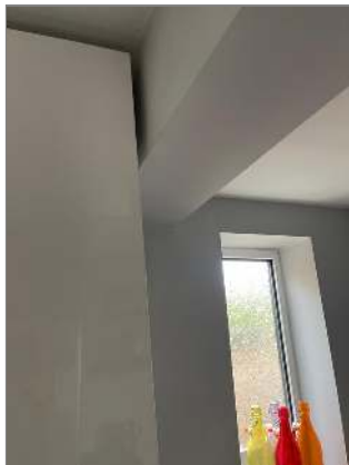
Photo - 93 Rear opened up - kitchen to cloaks
