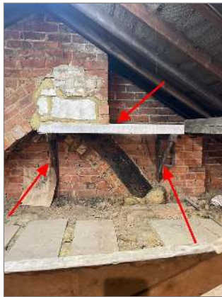
Photo - 66 Support for chimney breast
