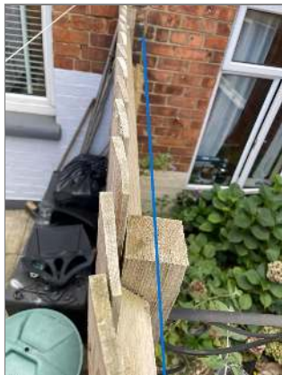
Photo - 156 Correct boundary line?
